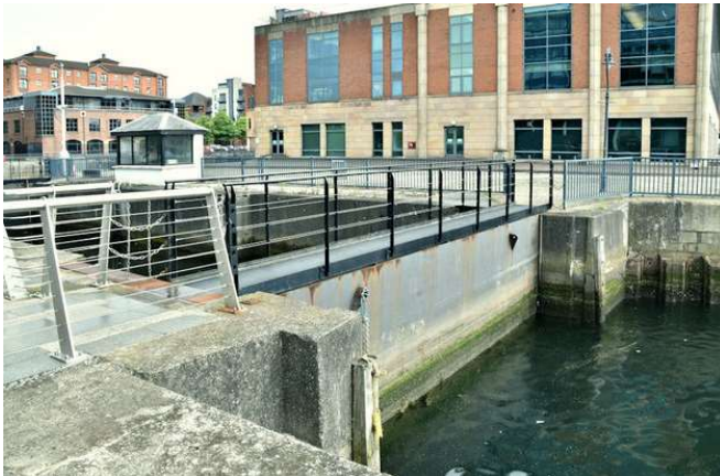
Figure 6: Pinch point, Barrier 20
